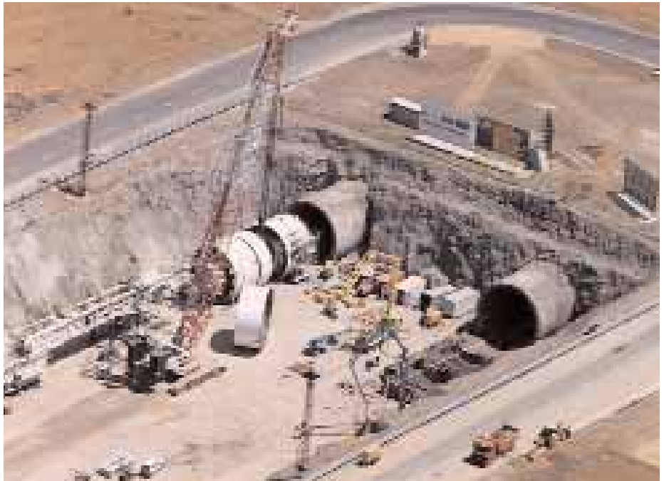
■ Guadarrama tunnels. Madrid
