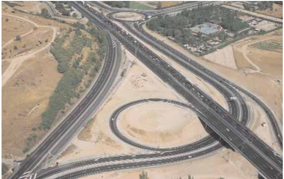
■ Connection of the M-50 with the A-1 relief road. Algete junction. Madrid
