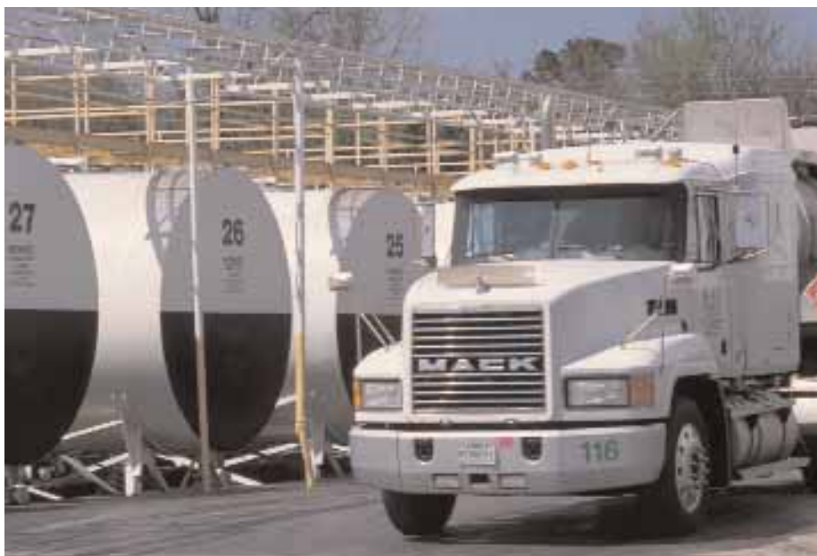
■ Wastewater treatment plant in South Carolina. USA.
