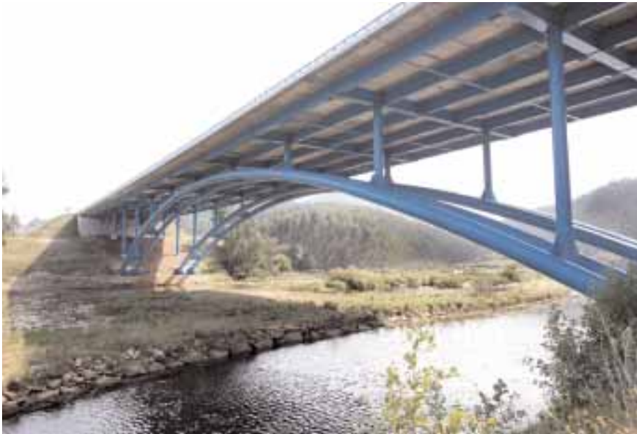
■ Viaduct over the Escudo River. Cantábrico dual carriageway
