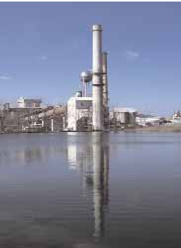
■ Cement factory in Keystone. USA
