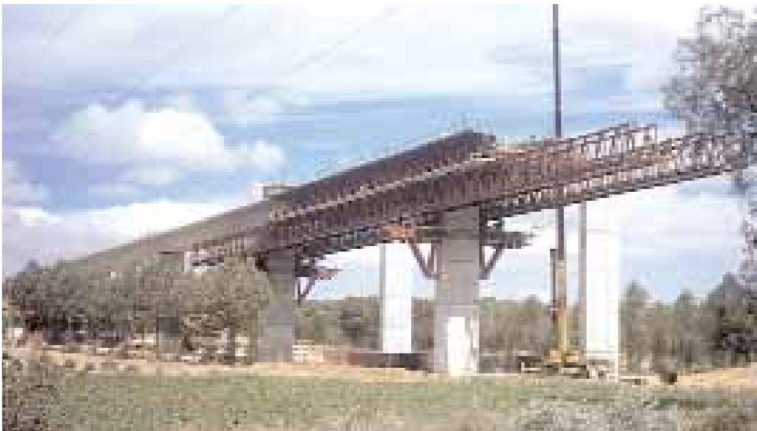
■ A-11 Duero dual carriageway. Toro-Zamora section. Viaduct over the Adalia Stream
