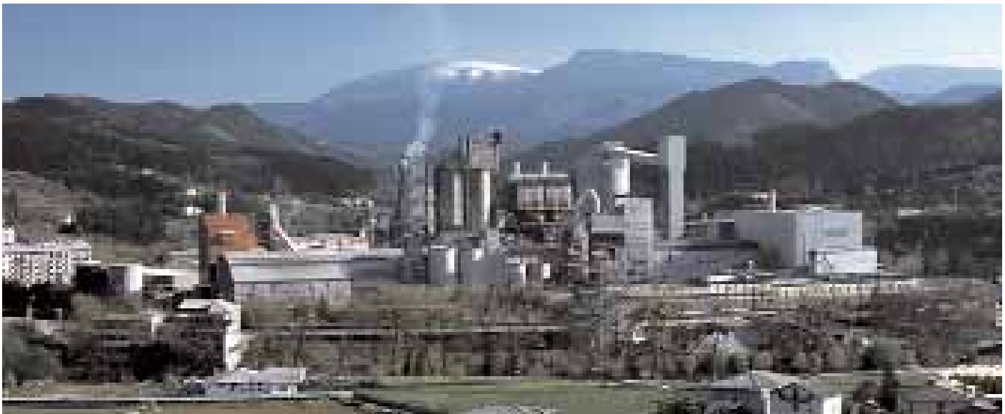
■ Cement factory in Lemona. Vizcaya
