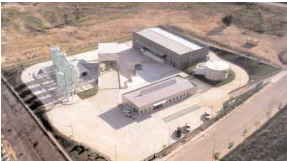
■ Industrial waste treatment plant in Valdebebas. Madrid
