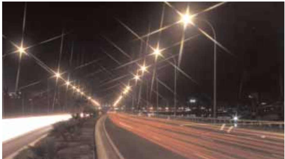
■ Lighting of the R-3 arterial road. Madrid
