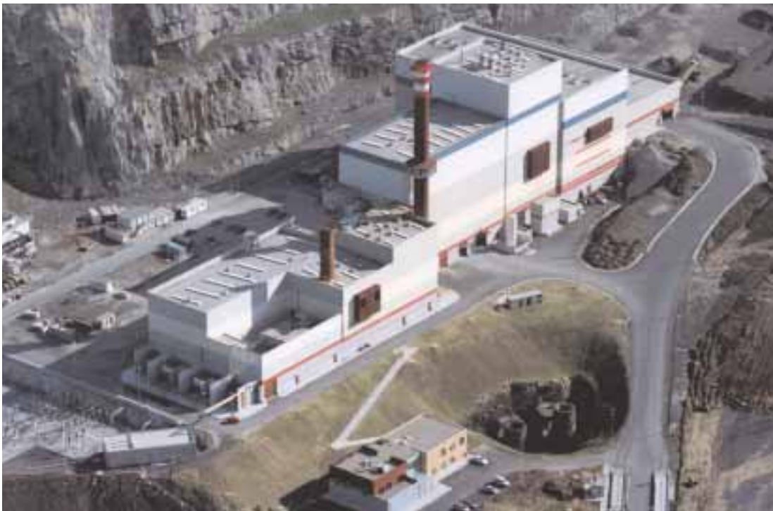
■ Solid waste treatment plant in Zabalgarbi, Vizcaya
